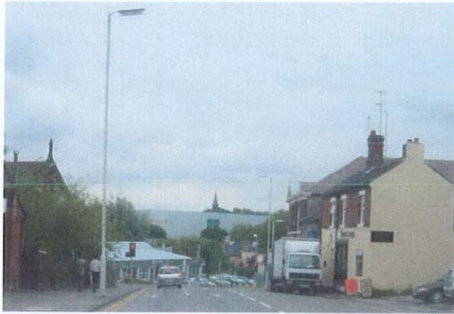
Photograph 4.4: Approach to the traffic signals at A525 – Pooldam
